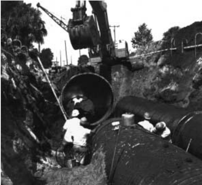
Smooth-lined CSP storm sewer being installed.
