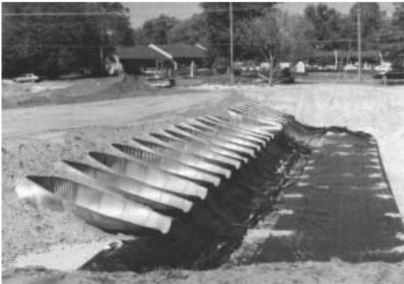
A "Toys R Us" facility in Ocala, FL during construction showing a detention basin constructed of 18 lines of 1200 mm (48 in.) diameter fully perforated corrugated steel pipe used for a recharge system.
