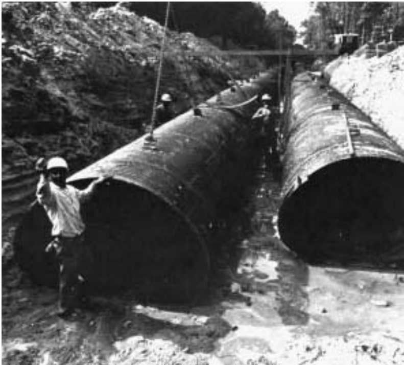
Storm Sewer installation involved 1300 m (4300 ft) of full bituminous coated full paved pipe arch.
