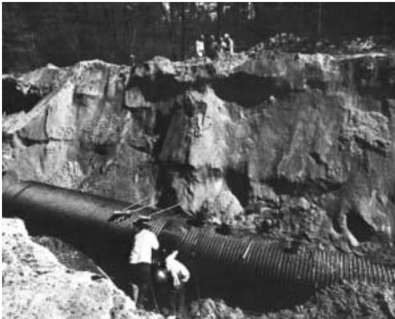
Standard CSP structural designs permit unrestricted trench width.
