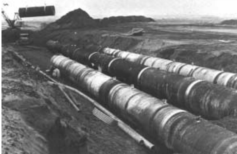
3000 mm (120 in.) diameter, 75 x 25 mm (3 x 1 in.) prefile full bituminous coated and full paved; 1500 m (5000 ft) installed as stream enclosure for runway extension.
