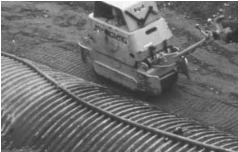
Adequate, uniform compaction is the secret to building soil and steel structures.
