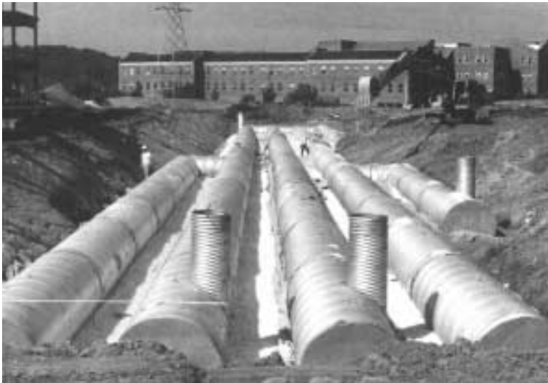
An example of a combination underground detention chamber and recharge system. Five lines of 1800 mm (72 in.) diameter corrugated steel pipe with 150 mm (6 in.) slots in the invert.
