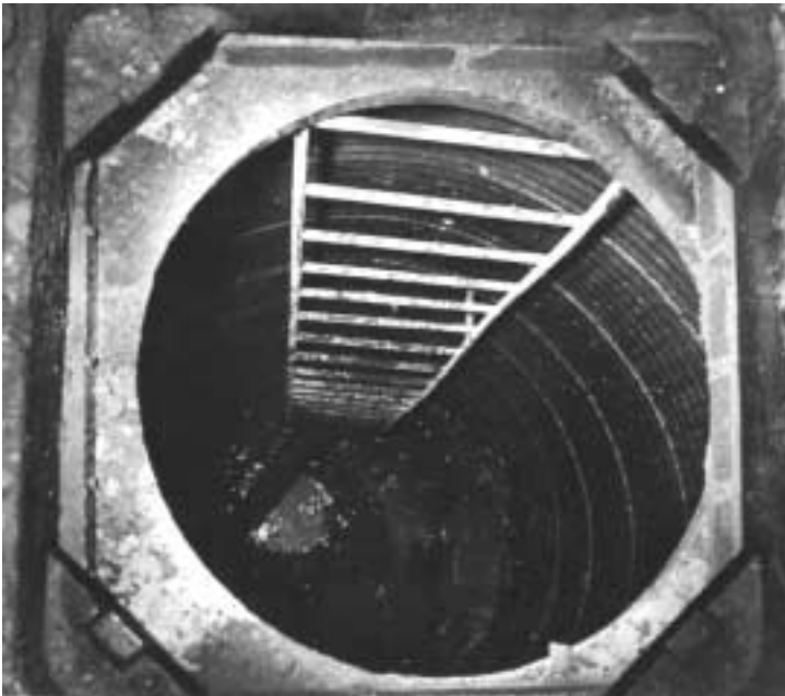
CSP catch basin with concrete slab and standard cast-iron frame and cover.
