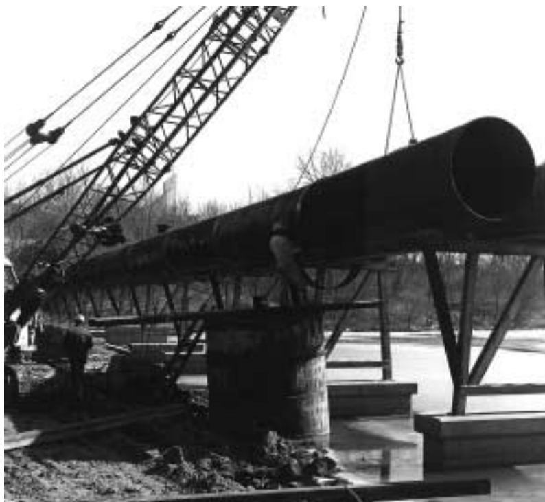
CSP aerial sewer being installed.
