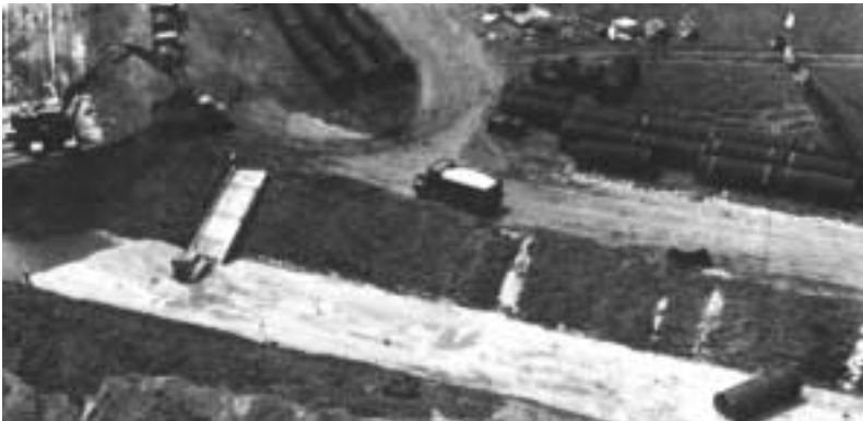
Philadelphia Airport, fiber-bonded, full bituminous coated and full paved CSP with semi-corrugated bands with O-ring gaskets, provides storm drainage for airport— 5800 m (19,000 ft) of 2100 mm (84 in.) through 2550 mm (102 in.) diameters, 2-3 m (6-10 ft) of cover.
