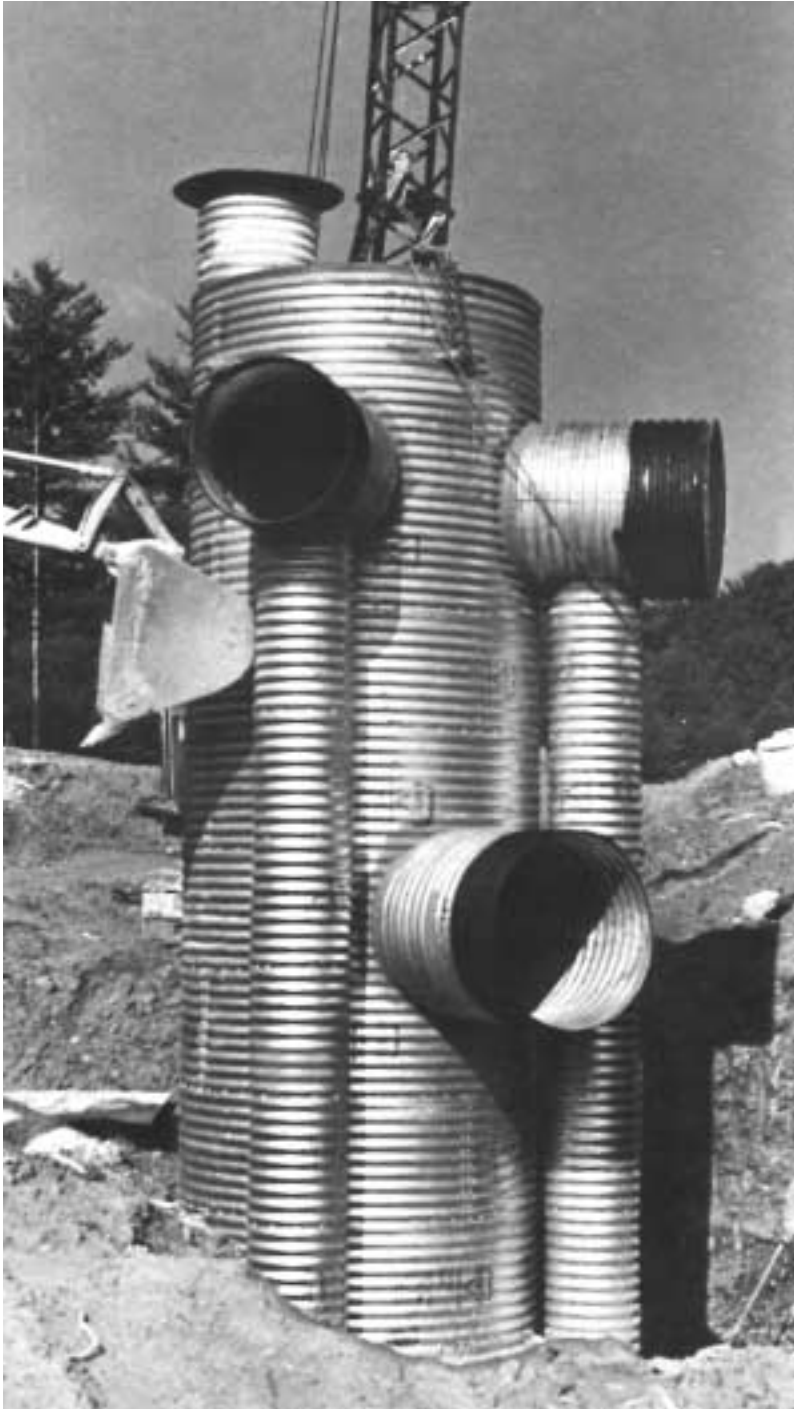
Fabricated fittings can be made to solve almost any sewer problem.
