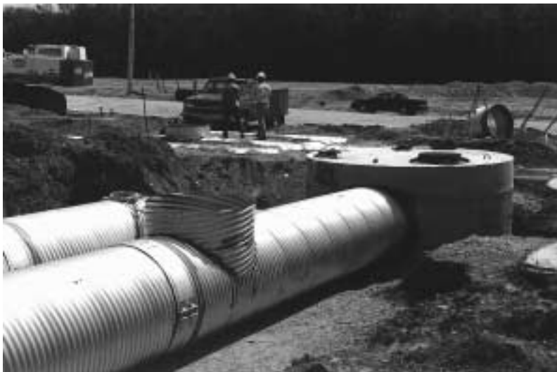
Recharge trench installation showing junction box.
