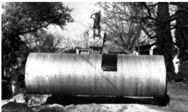
Installing a fully paved sanitary sewer.
