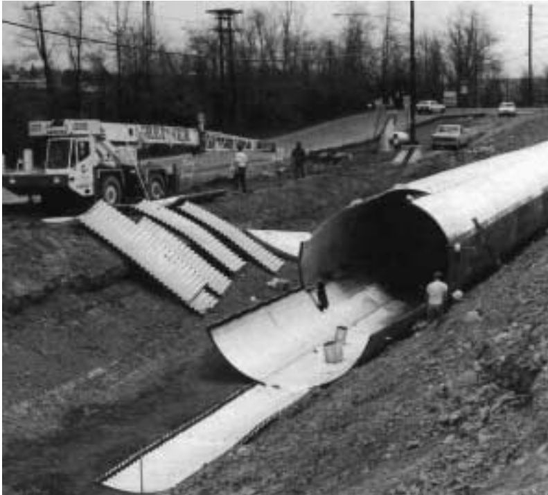
100 m (320 ft) of 3825 mm (12 ft - 5 in.) diameter structural plate pipe with gasketed seams used as an underground detention chamber collecting runoff from a shopping center near Harrisburg, PA.
