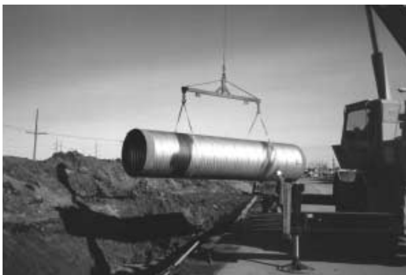
Exterior coatings are protected during installation by use of lifting lungs or slings.
