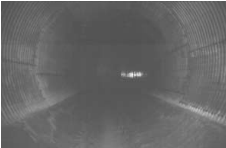
Concrete inverts can solve abrasion problems.
