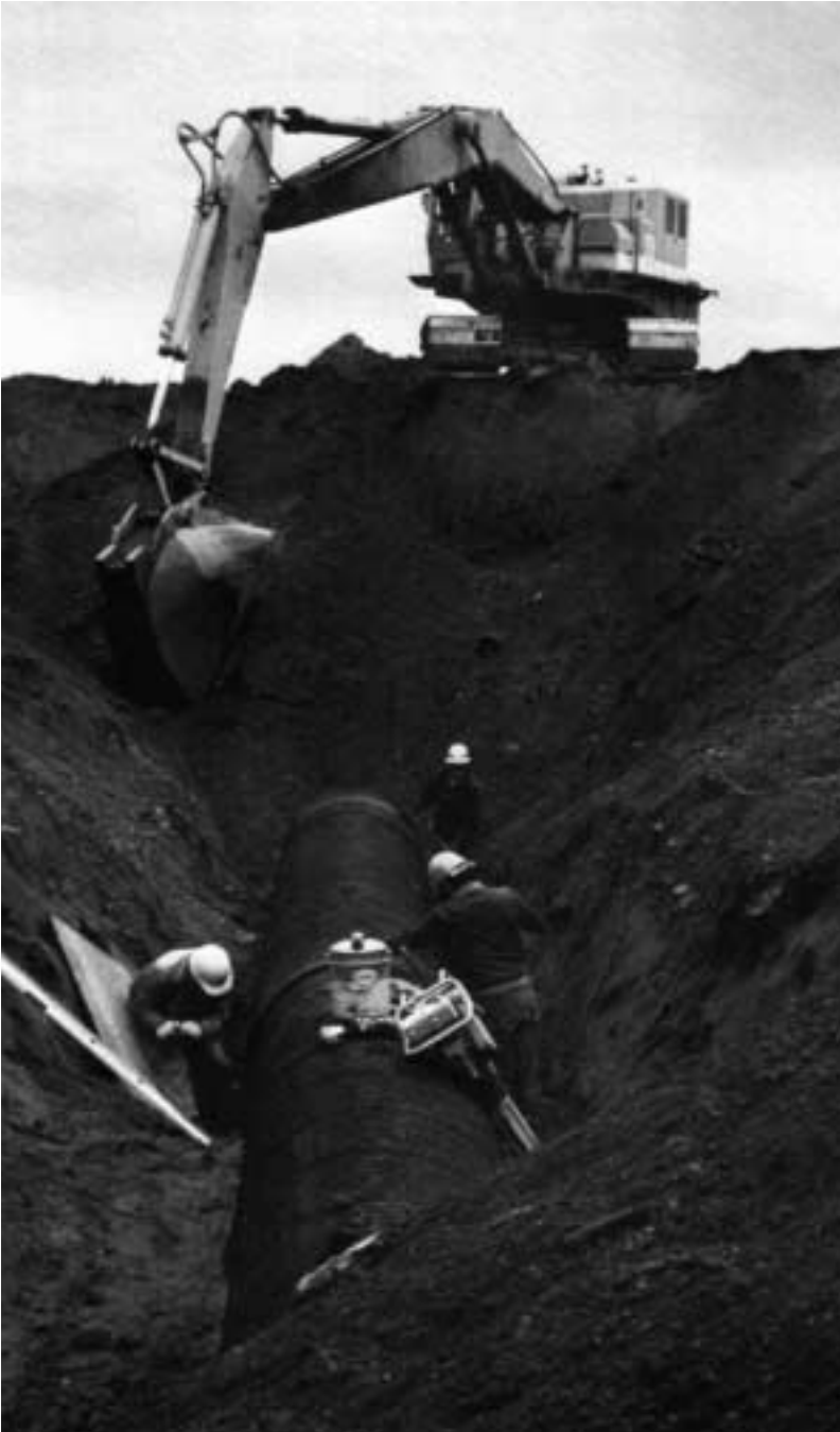
CSP sewers are designed for the deepest installations.
