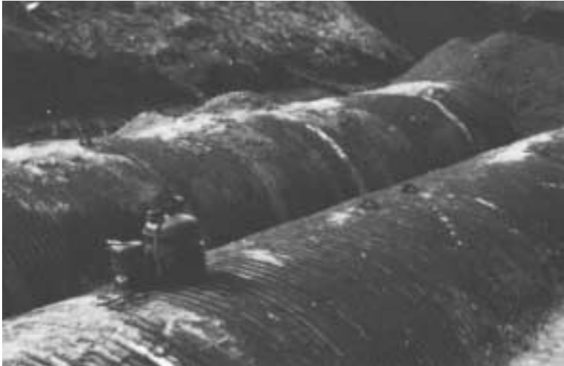
Philadelphia Airport expansion again calls for CSP storm sewers. Corrugated steel pipe was installed 25 years before in an earlier expansion.
