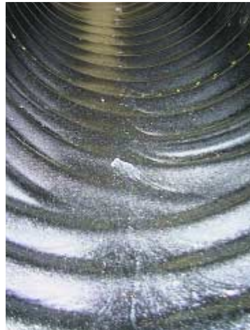
FIGURE 6. Polymerized asphalt over galvanizing after test run 3.
