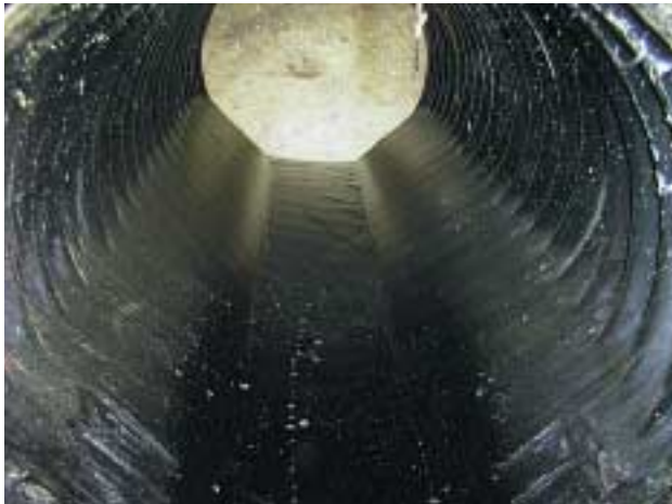
FIGURE 5. Asphalt paved pipe after test.
