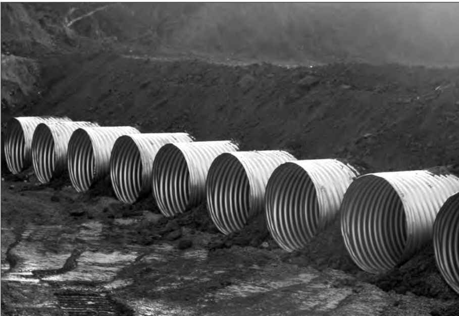
■ Multiple lines of CSP provide an effective low profile culvert crossing.
