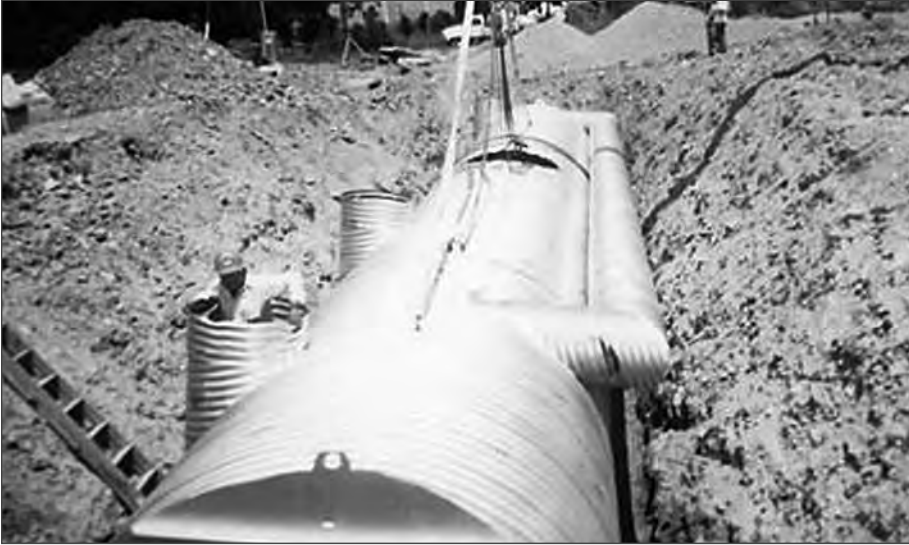
■ Effective water quality is attained by using an underground CSP sand filter.
