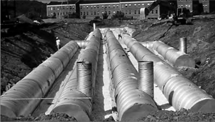
■ Typical CSP underground detention system.
