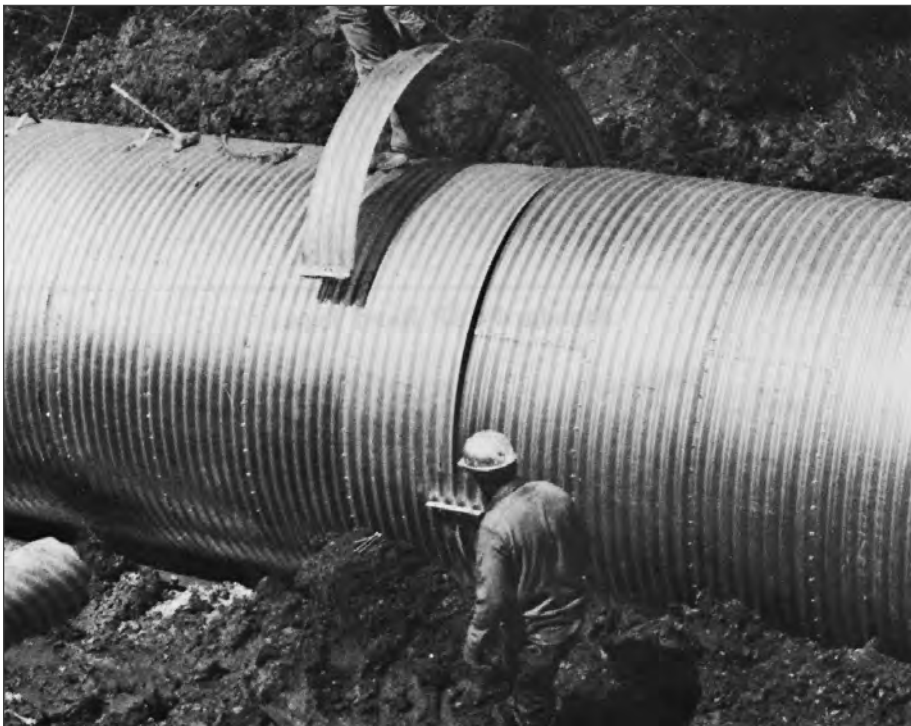
■ Two-piece corrugated band joins length of annular riveted pipe.
