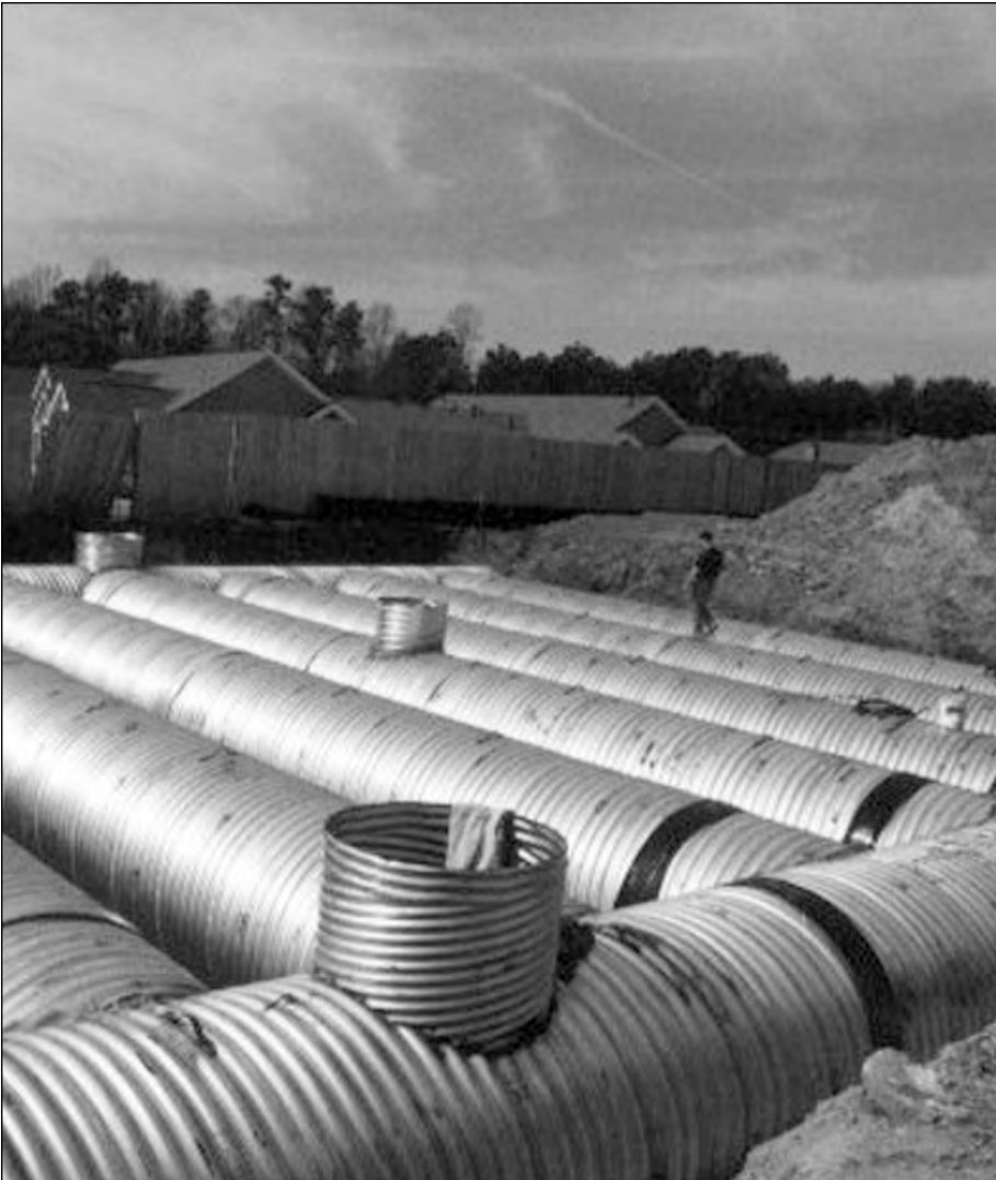
■ Typical CSP underground detention system for a new housing development.
