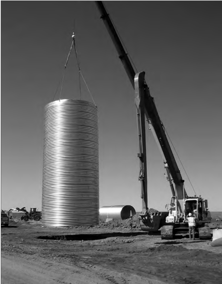
■ CSP form for wind turbine generator footing.
