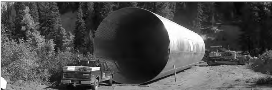
■ Fish Passage Project on the Mc Cloud River under the Mc Cloud Rail Road in Northern California. 16 foot and 20 foot diameter structural plate pipes.
