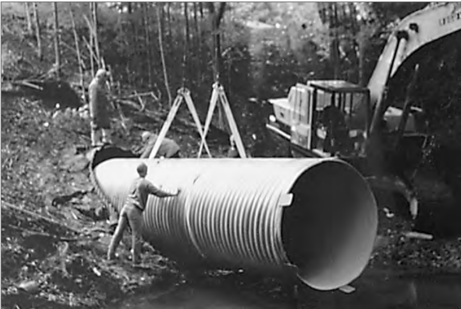
■ Figure 12.19 Slip lining with CSP.
