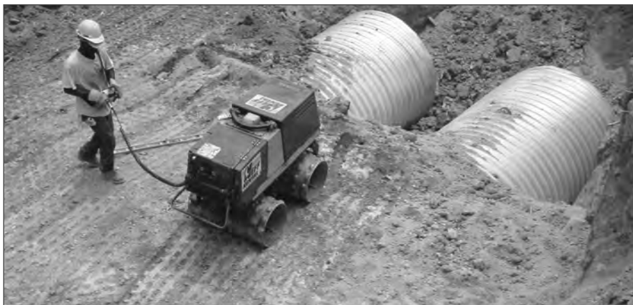
■ Figure 10.1 Proper compaction equipment close to structure.
