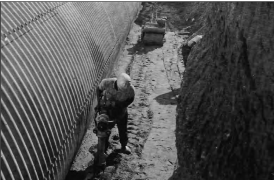
■ Figure 10.22 Proper use of Compaction Equipment.
