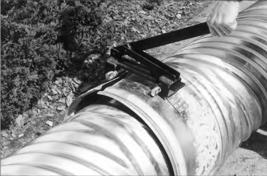
■ Figure 10.15 Band used to join reformed end helical pipe.
