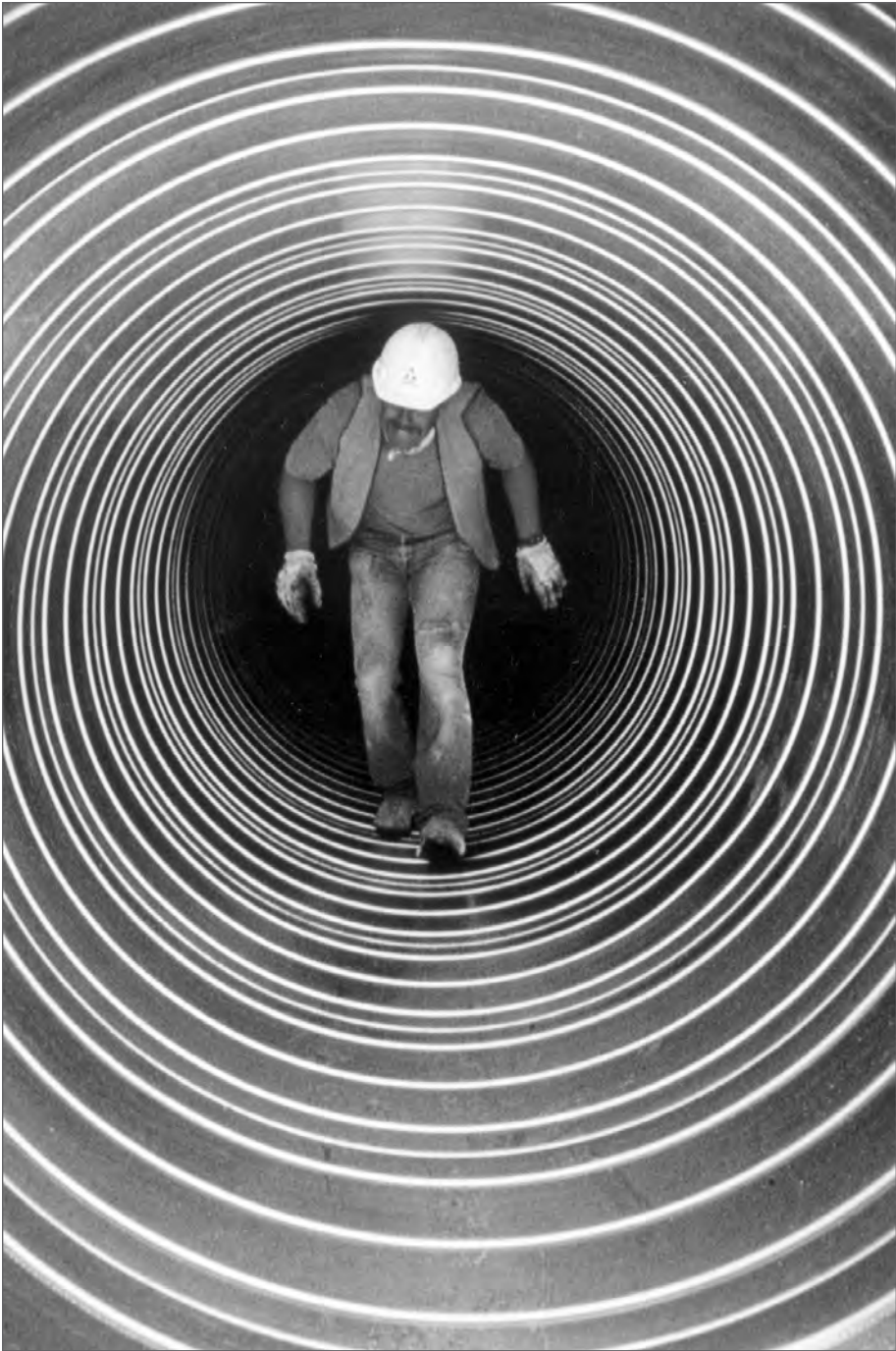
■ Figure 12.1 Pipe inspection.
