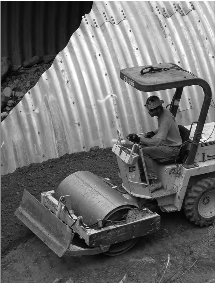
■ Proper backfill and equipment are important for a successful installation.
