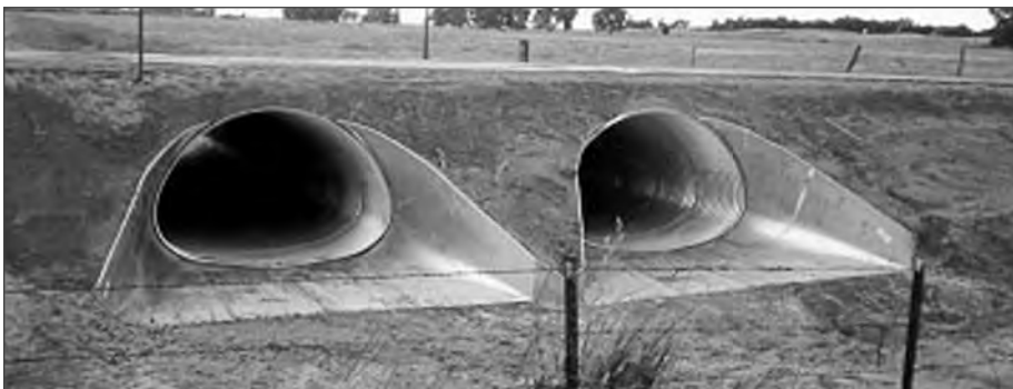
■ Figure 10.30 Corrugated steel pipe arch flared steel end sections.
