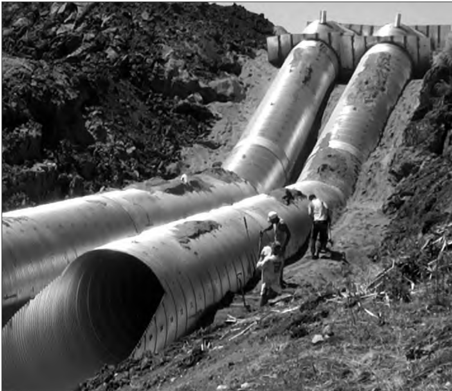
■ Installation of a corrugated steel pipe spillway. Note the anti-seep collars on the pipe.
