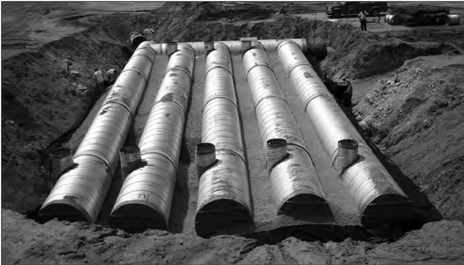
■ CSP underground detention.
