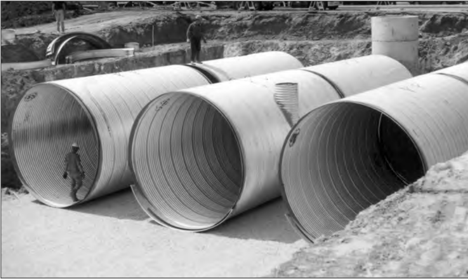
■ Typical CSP underground detention system being installed.
