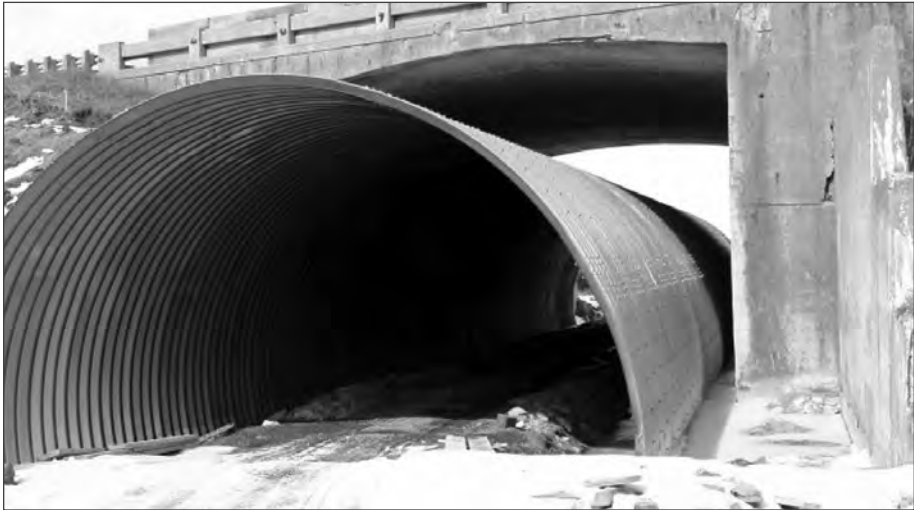
■ CSP bridge replacement provides an economical installation with short road closure time.
