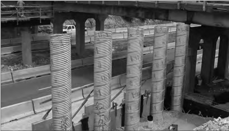
■ Bridge bent protection.
