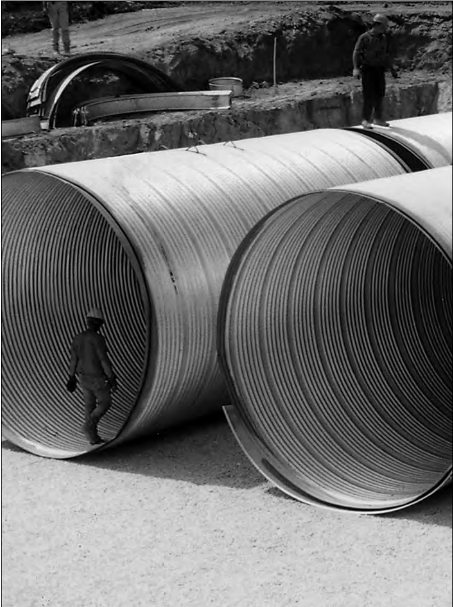
■ Typical CSP underground detention system.
