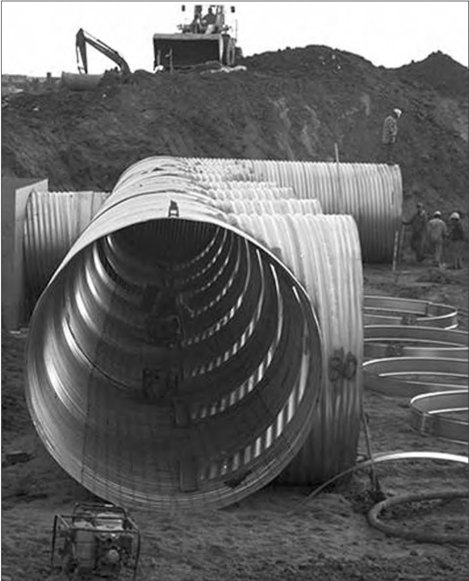
■ CSP underground detention system being installed.
