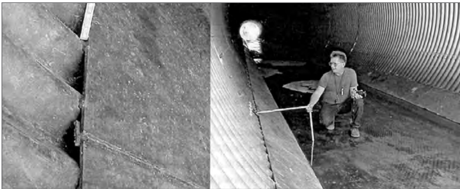
■ Figure 12.16 Steel armor-plated invert.
