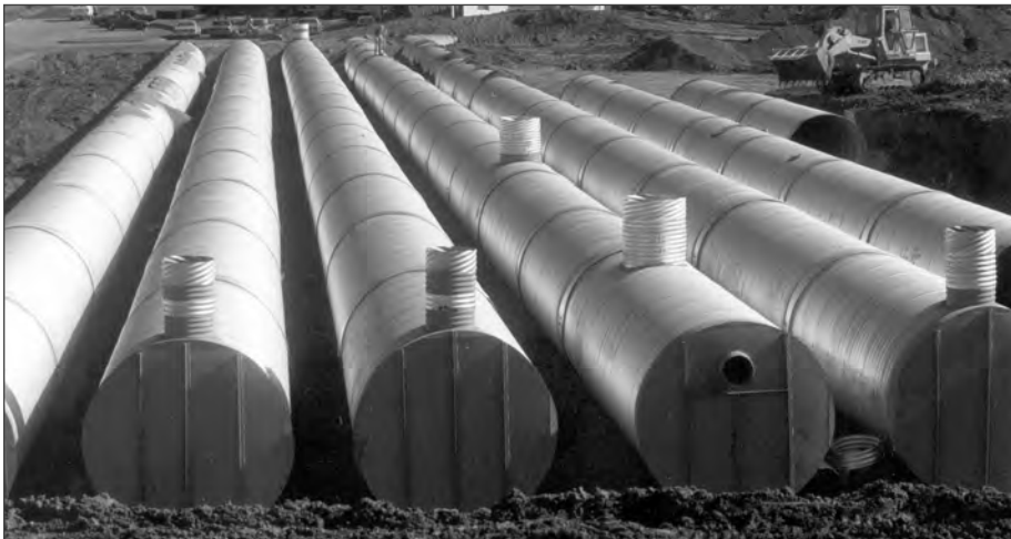
■ Shop attached CSP reinforced bulkheads.
