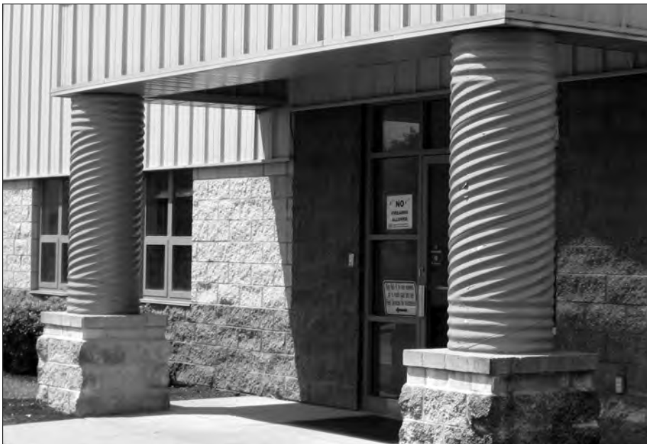
■ CSP entry columns for commercial building.
