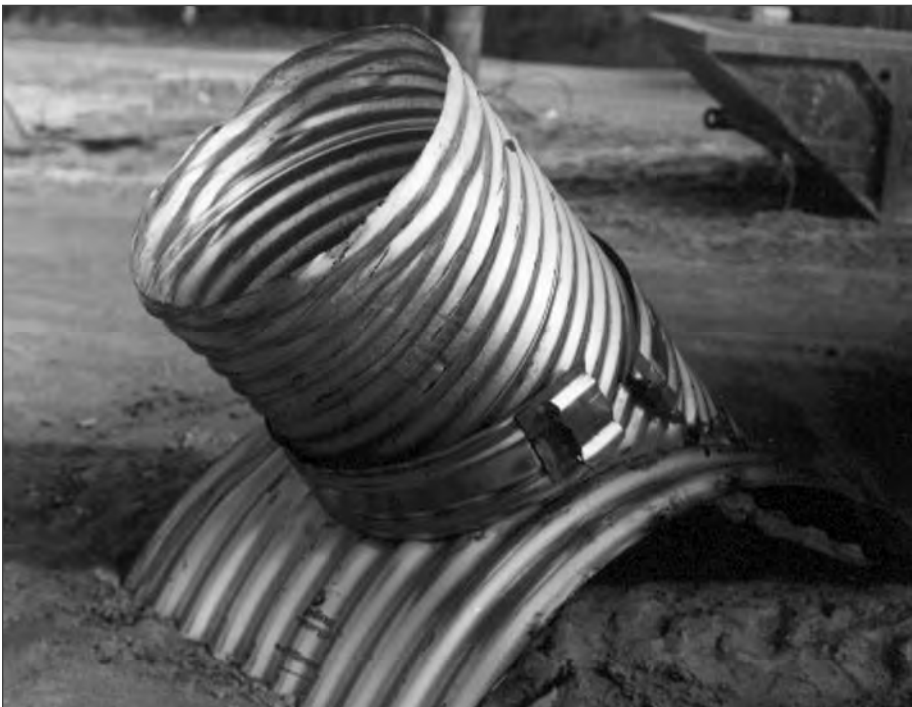
■ Figure 10.18 Typical CSP saddle fitting.
