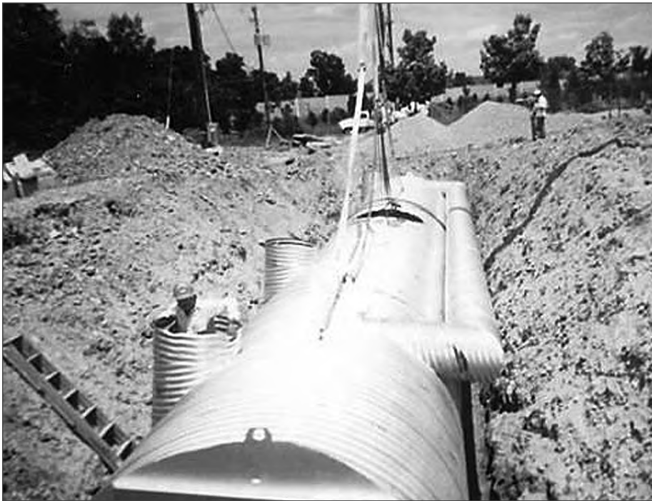
■ CSP sand filter system
