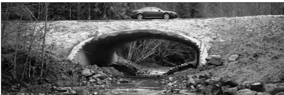
■ 36 foot span by 10 foot 5 inch rise deep corrugated box culvert with beveled ends, used for a Fish Passage project in the Willamette National Forest in Oregon.
