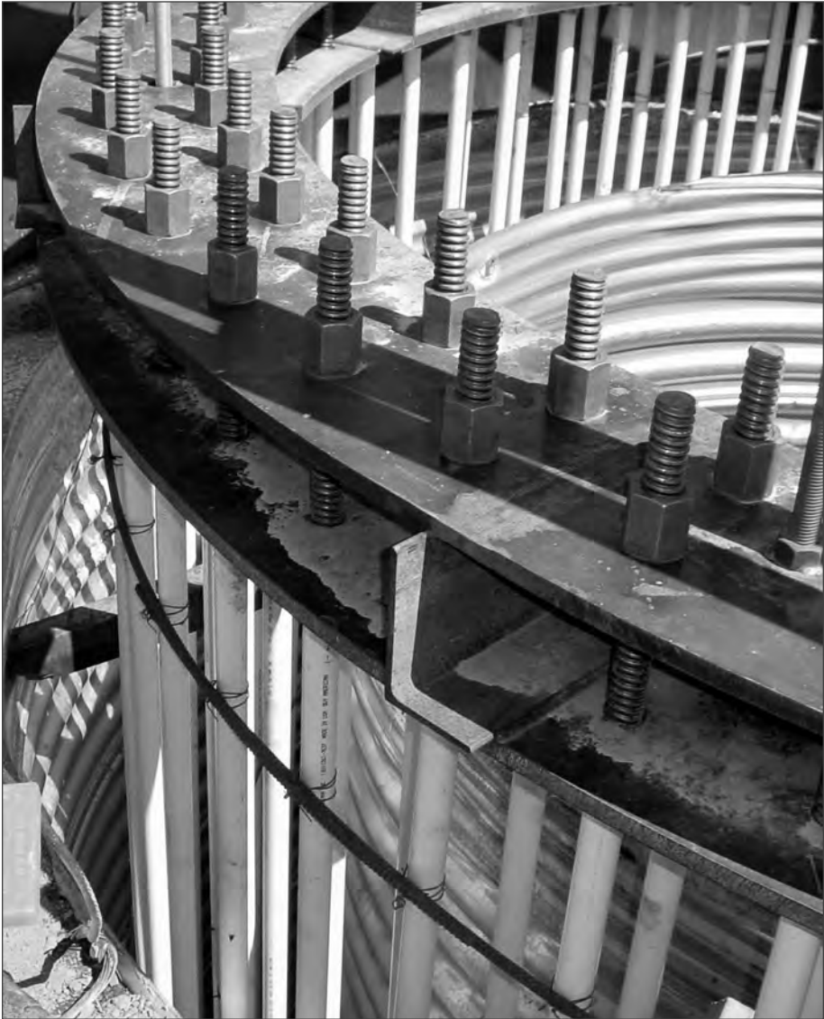
■ CSP form for wind turbine generator footing.
