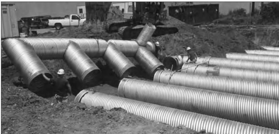
■ Typical CSP underground detention system.
