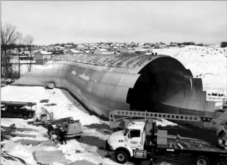
■ Figure 7.1 A corrugated steel long span structure will soon be a stream crossing under a freeway.
