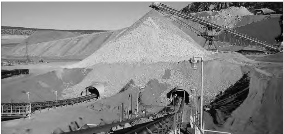
■ Structural plate pipe used for stockpile tunnels at a copper mine in Utah.
