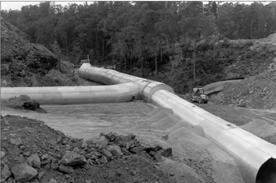
■ Figure 7.6 By far the most economical choice, this 19 foot diameter, corrugated steel structural plate storm sewer, using crushed rock backfill, carries 90 feet of cover.
