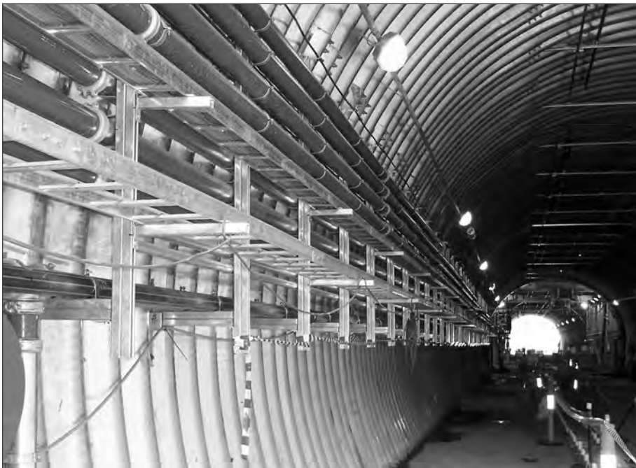
■ Corrugated steel utility conduit.
