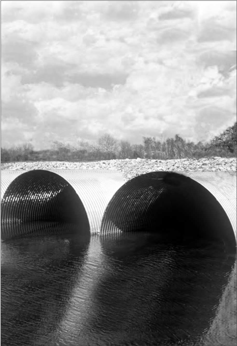
■ Round pipe multiple opening installation.
