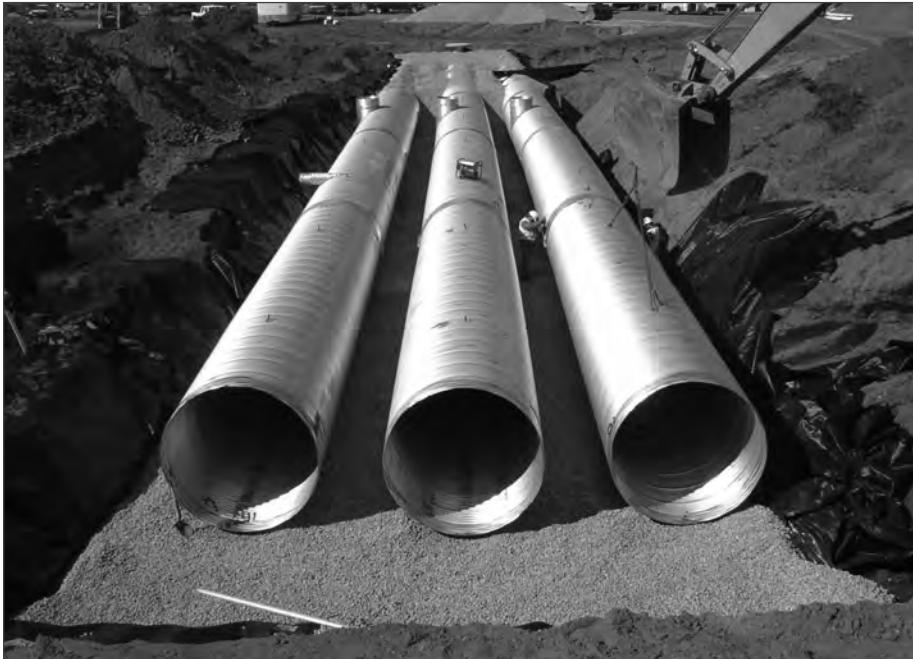
■ Figure 10.33 Detention system installation.
