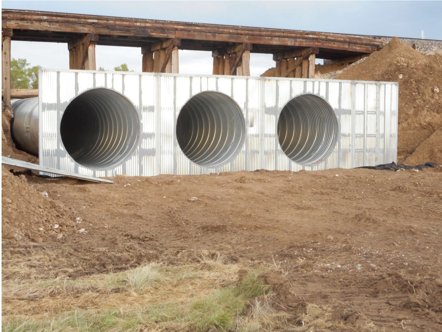
Rail Road Bridge Rehabilitation – Douglas Wyoming
