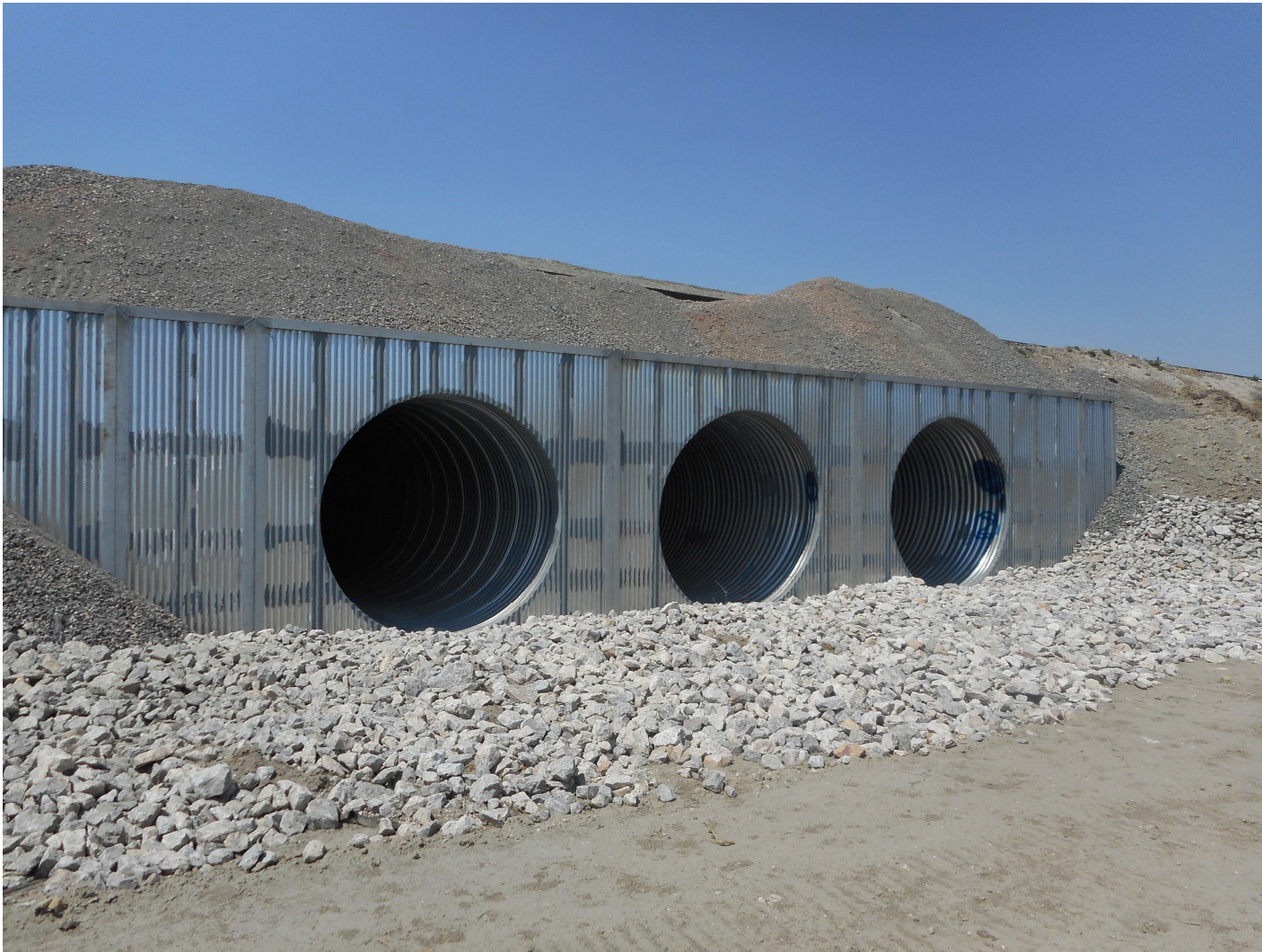
Rail Road Bridge Rehabilitation – Douglas Wyoming
