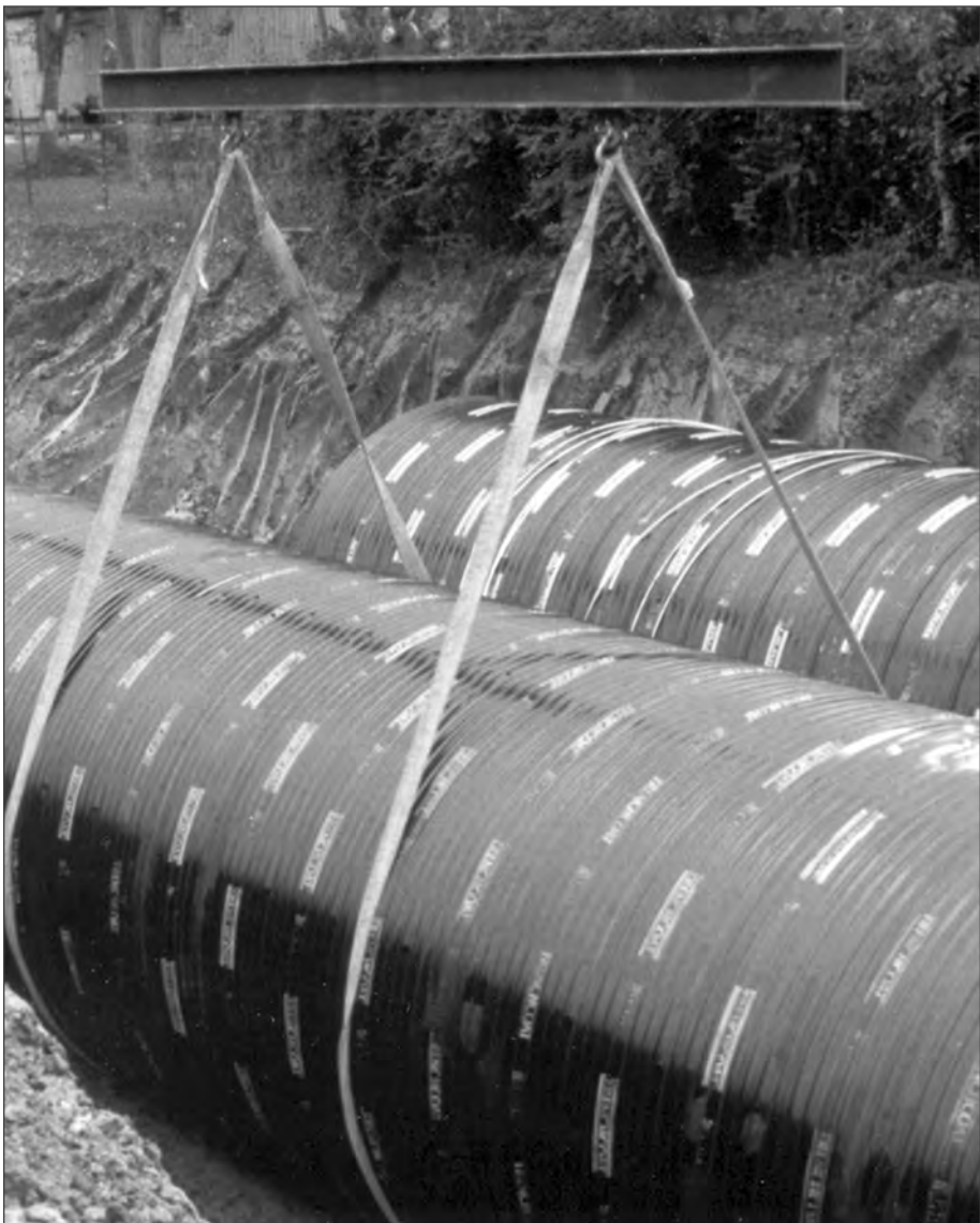
■ Installation of polymer coated CSP.
