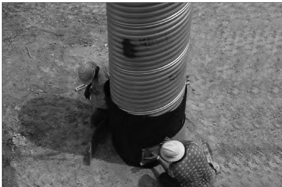
■ Figure 10.16 CSP manhole being installed.
