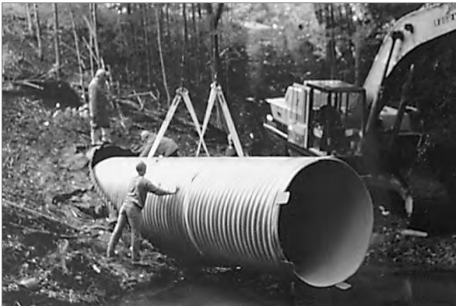
■ Figure 12.19 Slip lining with CSP.
