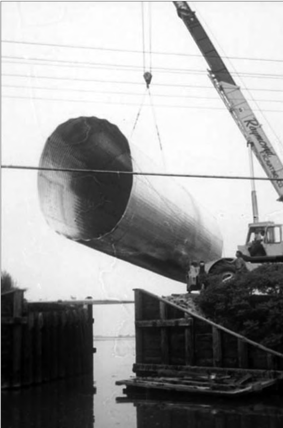
■ Figure 10.44 Assembled structure being placed in position.
