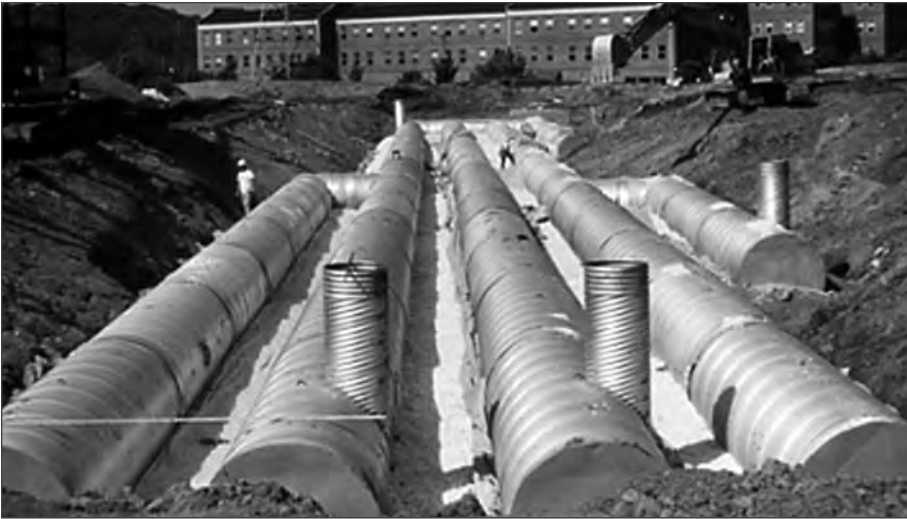
■ Typical CSP underground detention system.
