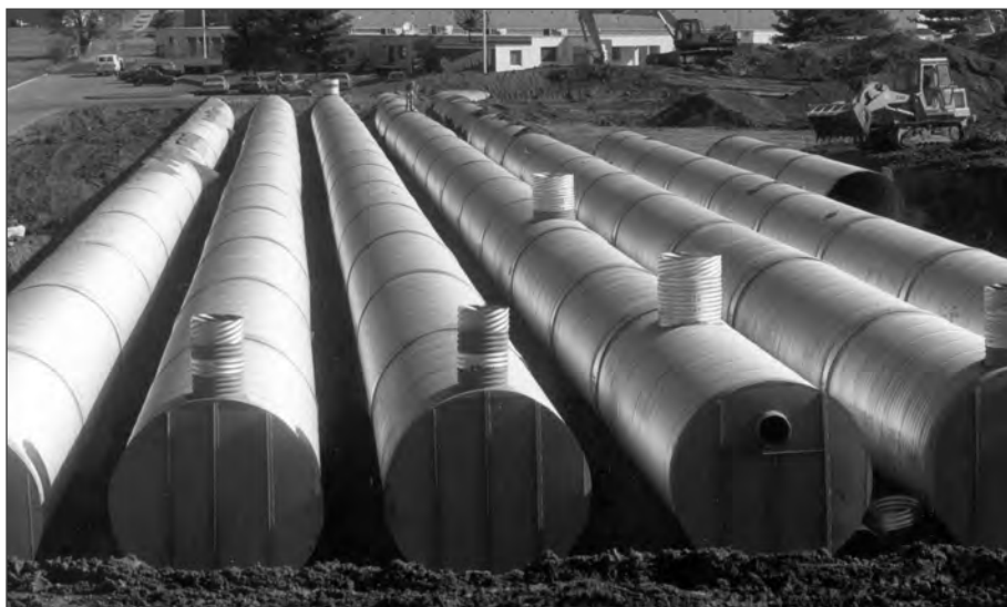
■ Site configuration adaptability and economical storage are accomplished with this detention system.
