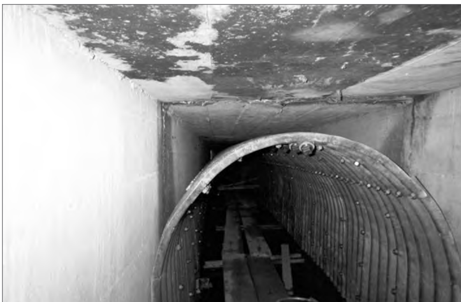
■ Figure 12.13 Structural plate arch with grout plugs used to line concrete box culvert.
