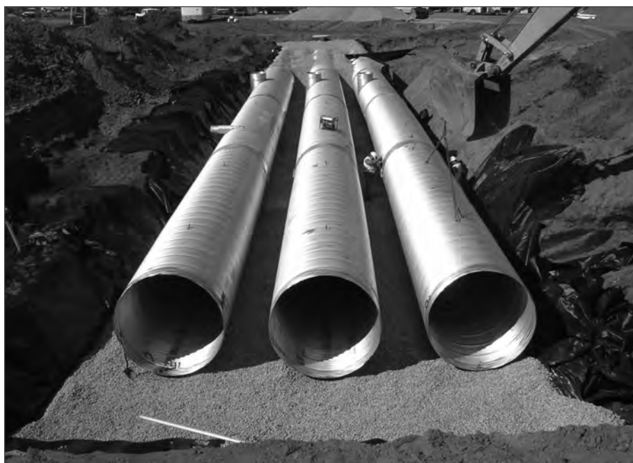
■ Figure 10.33 Detention system installation.
