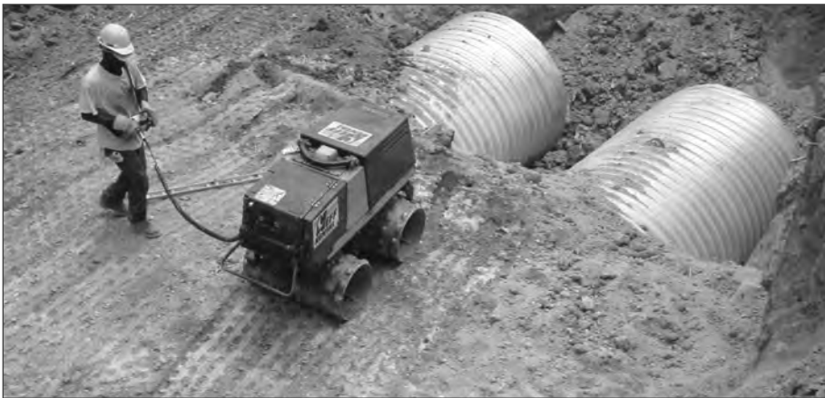
■ Figure 10.1 Proper compaction equipment close to structure.
