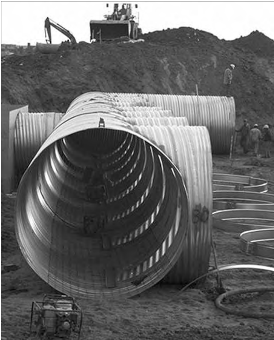
■ CSP underground detention system being installed.
