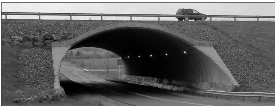
■ Figure 7.19 Long span grade separation.
