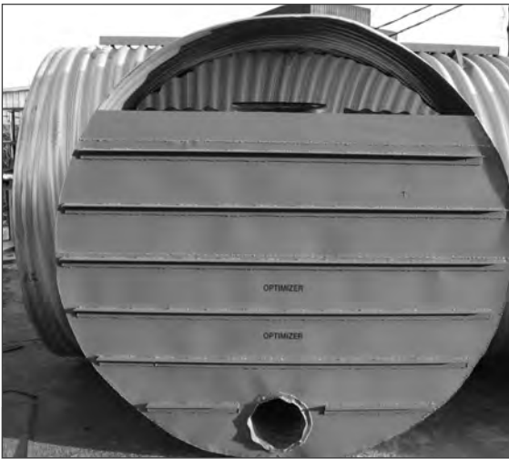
■ Internal CSP reinforced weir.
