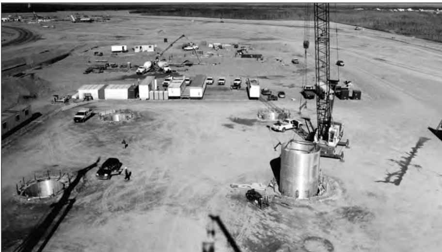
■ Inserting the structural plate shaft liner.
