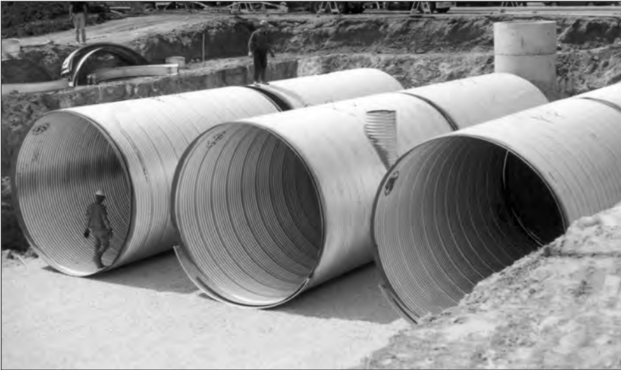
■ Typical CSP underground detention system being installed.
