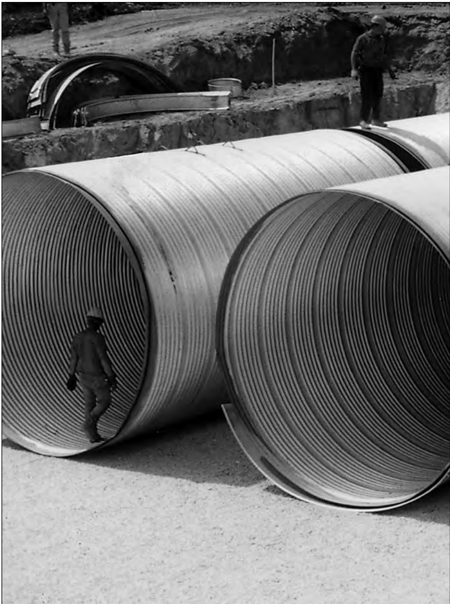
■ Typical CSP underground detention system.
