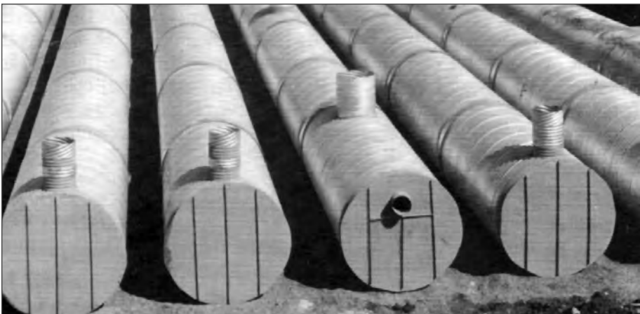
■ Figure 11.2 Seven lines of 96 inch CSP being installed to form an underground stormwater detention facility.
