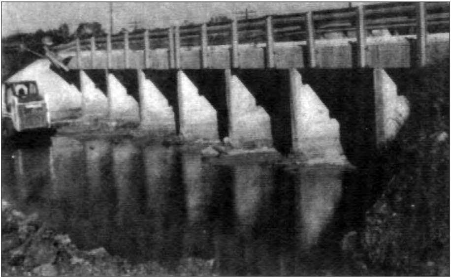
■ Figure 11.3 Texas DOT bridge replacement project. Before...
