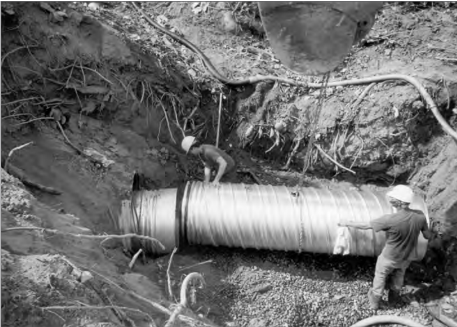
■ Figure 12.4 Pipe sections can be fabricated in lengths as required to suit slip lining installation.
