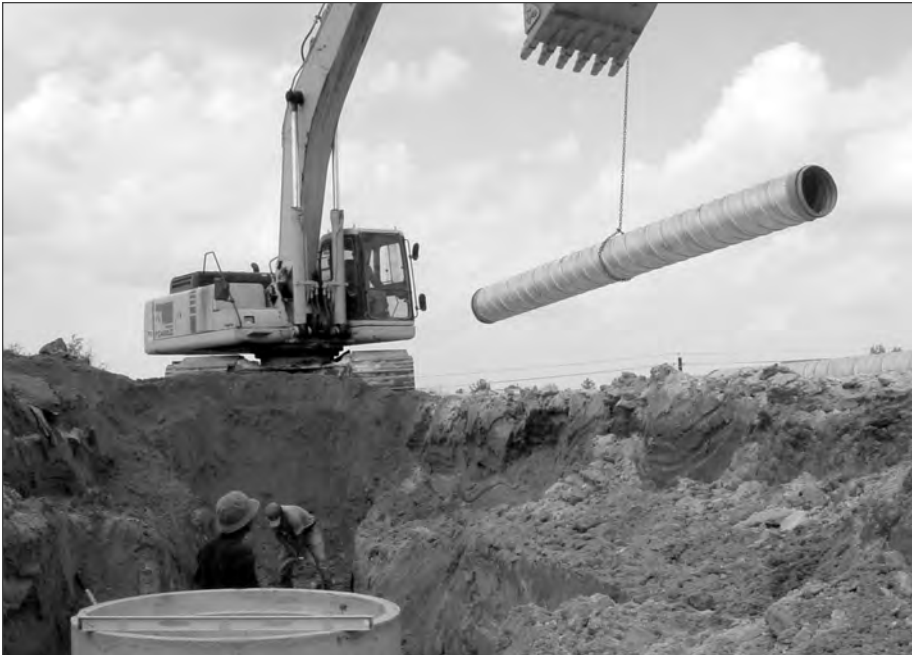
■ Figure 10.12 Lifting CSP into place.
