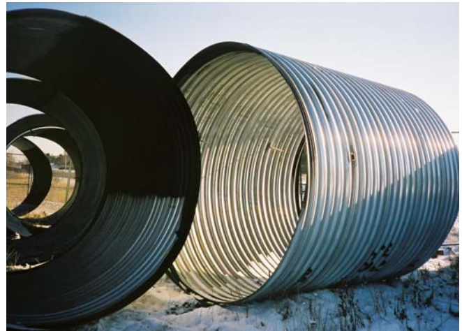
CSP with Screw Jacks and Grout Plugs
